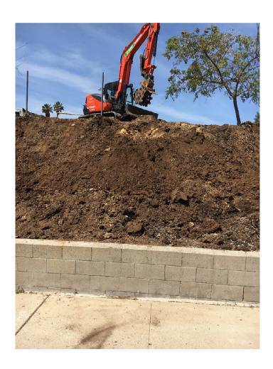
In January 2017, over 2" of rainfall occurred over the course of a few hours. The slope in front of Ladera school failed, and emergency work was undertaken to restore the slope.
